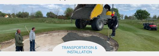
Crew moves wet mix to bunkers, levels at 2 inches and lightly rolls the surface
